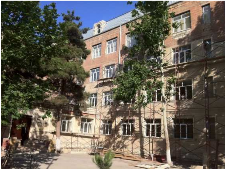
Vocational Lyceum No 2 in Ganja under reconstruction
