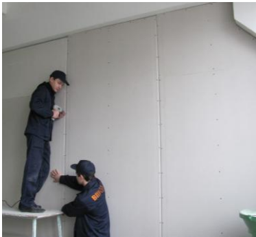
Installer of plasterboard structures
